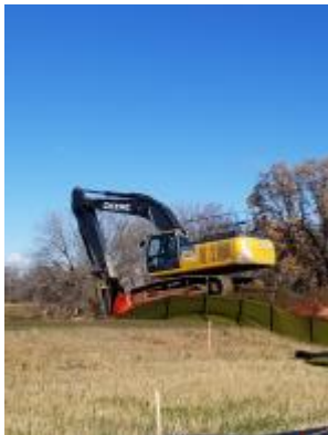
Excavator at Dead horse Creek Photo taken Northeast on South side of creek
