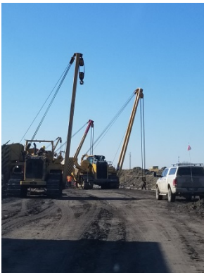
Lowering in and welding at SSKP 1054.179 (MB-WC71) Photo facing West
