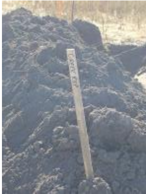
Separated spoil piles at 1054.179 Photo taken South
