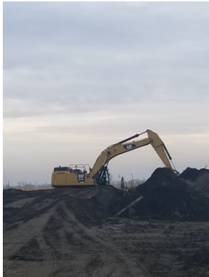
Excavator at 1054.200-(MBR-WC71) Restoring drainage. Photo taken facing East
