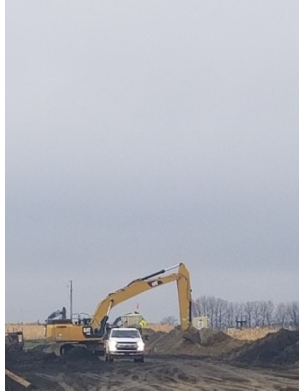
Excavator backfilling drainage 1054.200-(MBR-WC71) Photo facing West.
