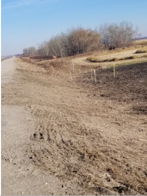
Harrowing bar ditch at Rd.7 Photo facing East
