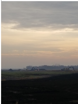
Rd.22 Final Clean up. Photo facing East
